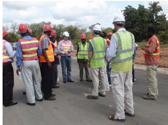
Mr. Mayock and Governing Board members getting brief on trial section of asphalt at km 9.300 + 9.400
