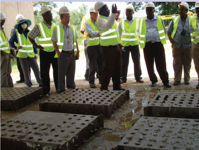
Eng. W.K. Christian MCA-T Director for Water projects providing details of the pre-casting of slabs for Water Rapid Sand Filter
