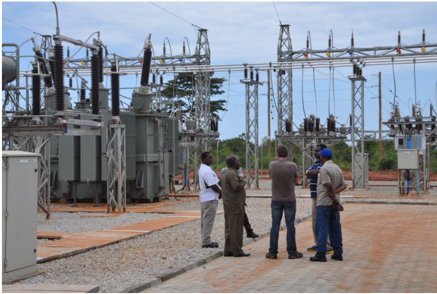
Visit at Kange substation 24 th October 2013
